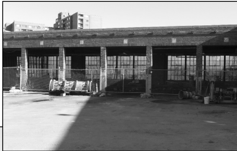
Interior and exterior views of the location today show overgrown, leaky, delapidated buildings which are no longer serviceable to garage the City's vehicles. (above:) Frozen water, leaking from the ceiling, now fills the pedestal sinks in the washroom. (below:) Most of the garage bays, with their "roofs of heavy plank" are fenced off as unsafe. (bottom:) Many of the large glass windows on the front are filled in. Others are broken.
