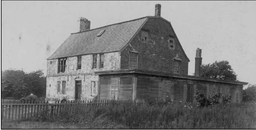
Peter Tufts House circa 1880 shows broken windows, no dormers, and an inappropriate single storey addition
